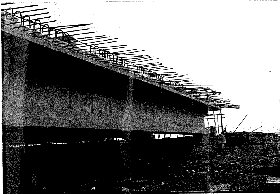
(a) Transversely post-tensioned bridge deck
